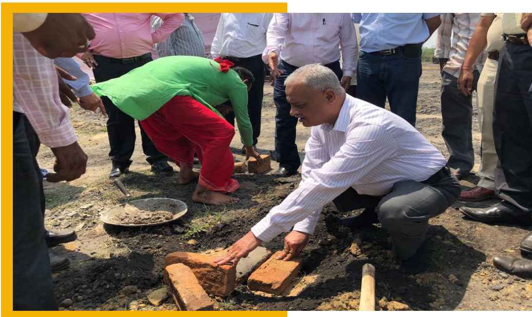
Bhumi Pujan at the Construction Site of 2.0 Mtpa Bhojudih Coal Washery by D(T)P&P and D(F).
